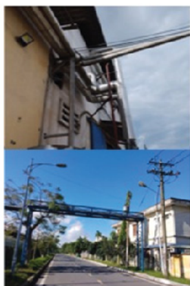
1. Steam pipe network connecting the three companies from the mutual boiler
